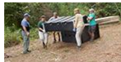
PVHC volunteers move a modular flotation component from the staging area to the wetland, where it will be assembled as part of the new floating bridge.
