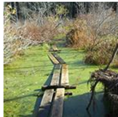
Before the 2016 project, hikers crossed the Rising Corner wetland on a narrow and deteriorating bog bridge.
