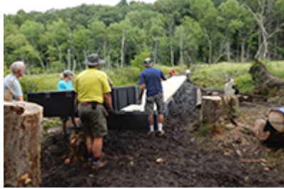
Section by section, the new floating boardwalk extended across the Rising Corner wetland as volunteers transported and positioned the modular components.
