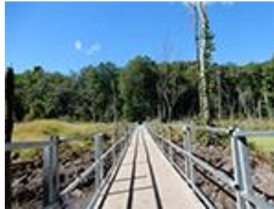
Completed in September 2016, the Rising Corner floating boardwalk carries MA Section 1 of the New England National Scenic Trail across the Southwick wetland.
