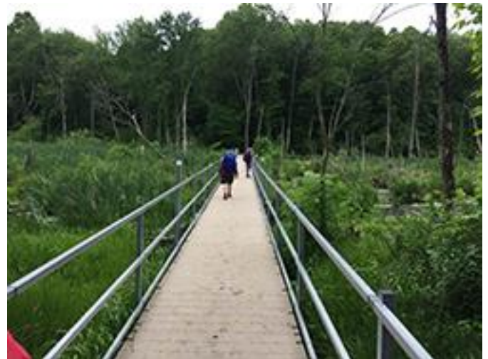
Bog bridge on Section I of the New England Scenic Trail in MA (photo by Rick Ricci)
