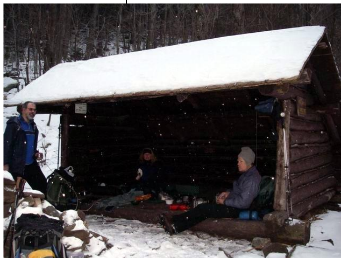
Batavia Kill Lean-to near Blackhead Mountain
