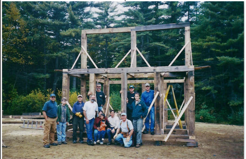
Shelter and Work Crew after First Weekend
